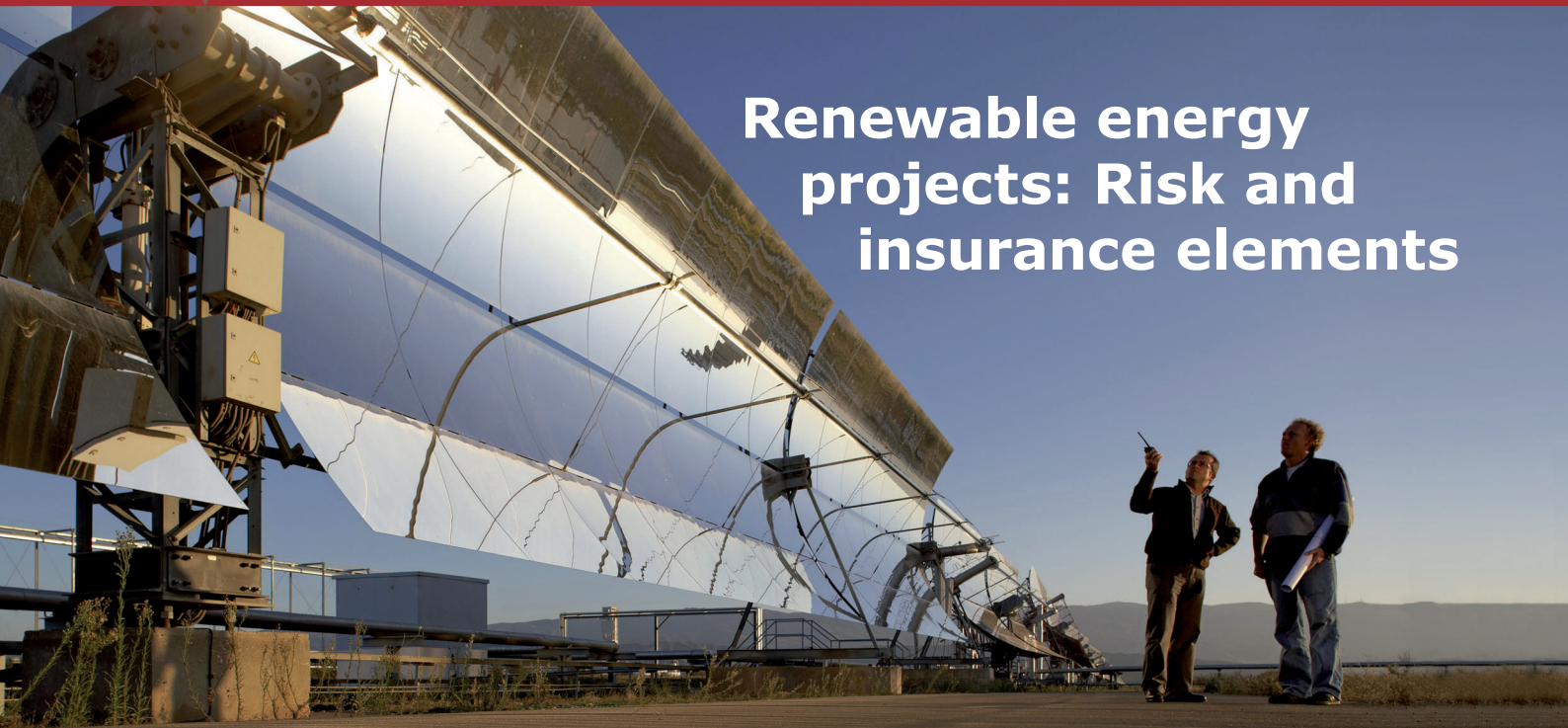
A parabolic trough power plant similar to the ones used in Masdar City (Photo: Hauke Dressler)
